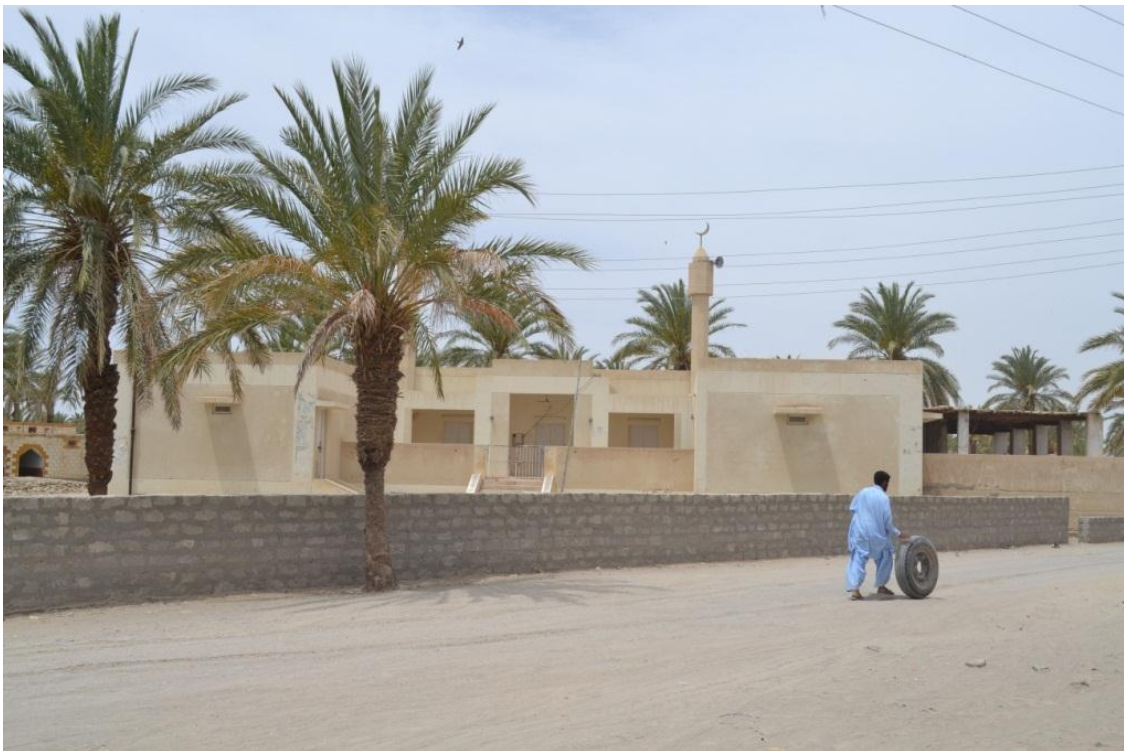
Fig. 5 View of a RC structure of a mosque in West Zawag
