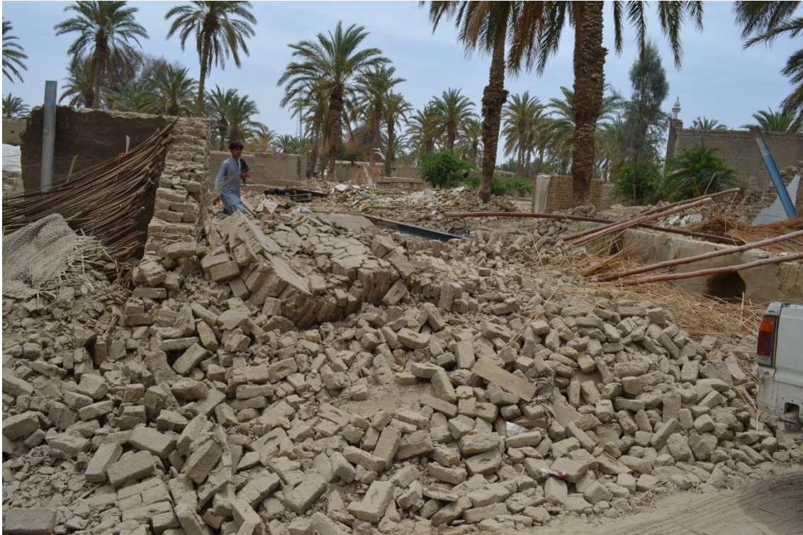
Fig. 8 View of damages in West Zawag
