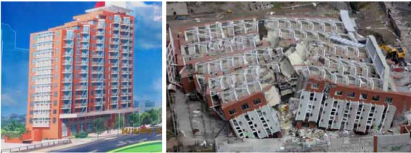
Figure 25. Collapse of tall building with discontinued structural wall at one corner (Concepcion, Chile, 2010; from Elnashai *et al*, 2010)
