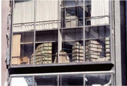
Figure 16. Excessive gravitational loads associated with change of use of building (Mexico City, 1985)
