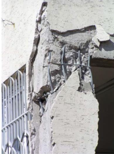
Figure 23. Failure at top of RC column, associated with poor reinforcement details (Bingöl, 2003; from Gur *et al*, 2009)
