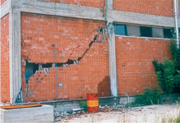
Figure 24. Two combined failure mechanisms for a masonry panel: diagonal tension both in panel and in confining frame (Adana-Ceyhan, Trukey, 1999; from Bachmann, 2003)
