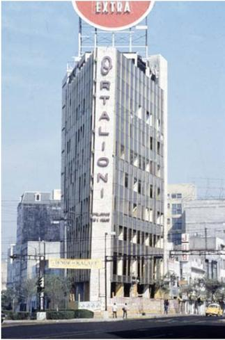
Figure 7. Pronounced asymmetry of stiffness (Mexico City, 1985)
