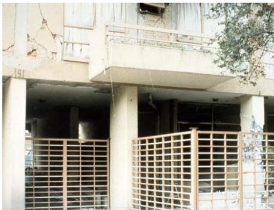
Figure 13. Weak-ground-story building with elevator core; compression failure of column due to overturning moment (Mexico City, 1985)
