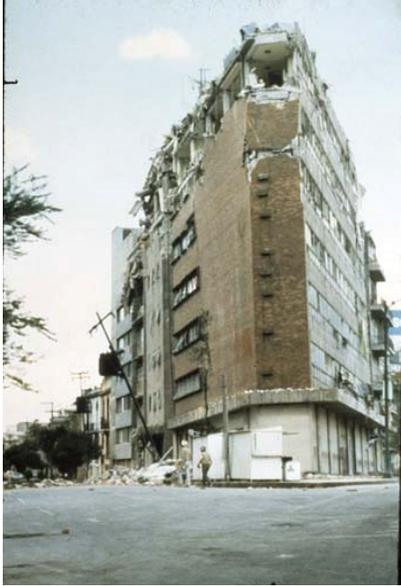
Figure 20. Upper story failures
