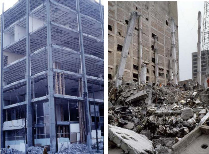
Figure 19. Typical waffle-slab multi-story building and collapse of a similar system (Mexico City, 1985)
