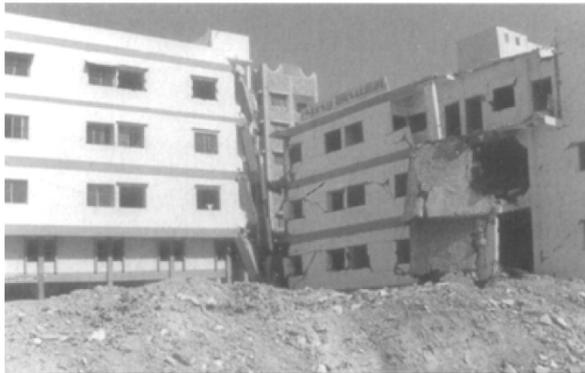
Figure 10. Collapse of weak ground story of building, with survival of upper stories (Gujarat, 2001; Murty *et al*, 2002)
