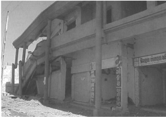
Figure 12. Partial collapse of one end of a long building with flexible floor diaphragms (Gujarat, 2001; Murty *et al*, 2002)
