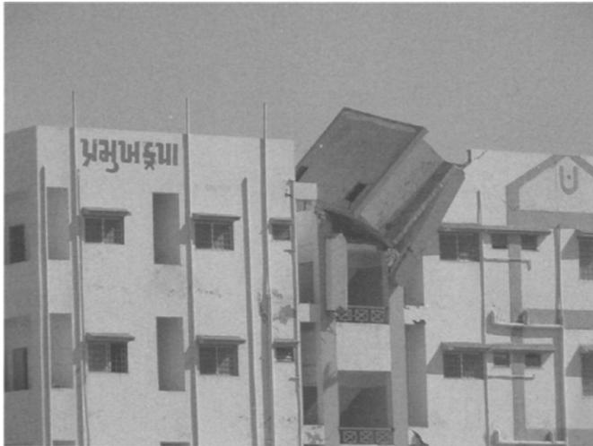
b) Collapse of water tank on top of RC building
